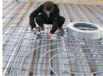
Laying underfloor heating/cooling pipes
