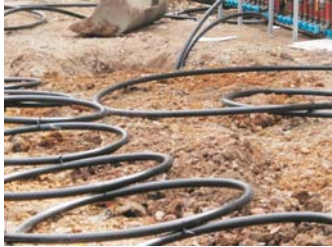
Ground source heat pump slinkies
