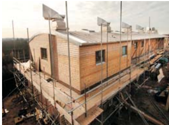
Hockney Green during the build process
