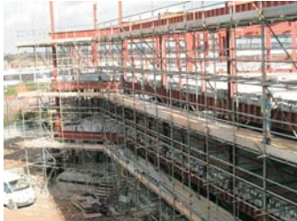
Exposed concrete assists with cooling and preheating
