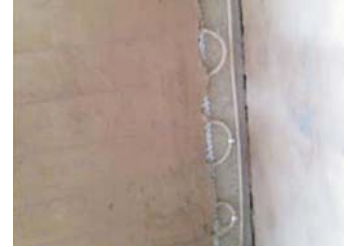
Plastered over insulation, with a mesh under the 2nd layer
