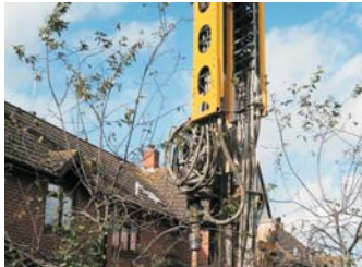
Drilling boreholes for ground source heat pumps
