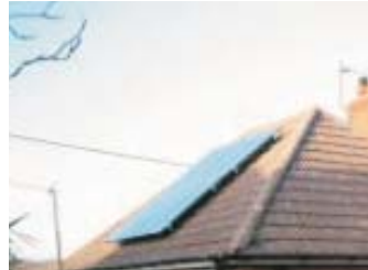
Refurbished houses with solar panels
